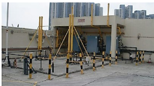
Buried LPG tanks supplying a metered facility
